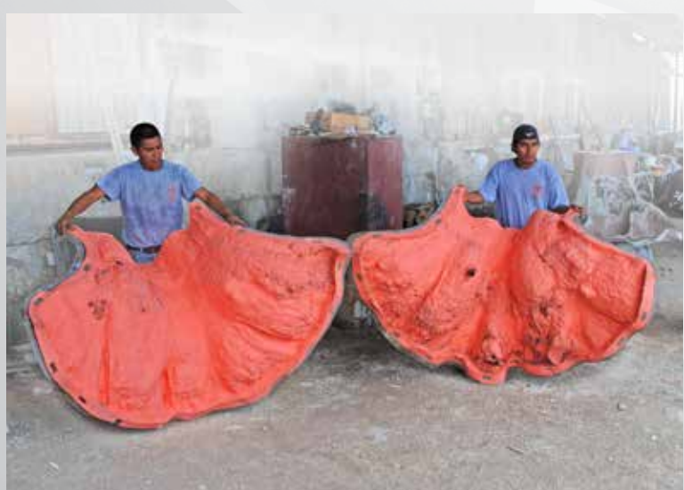
4 A support shell is applied, allowed to cure and then removed. The rubber mold is removed and ready for GFRC casting.
