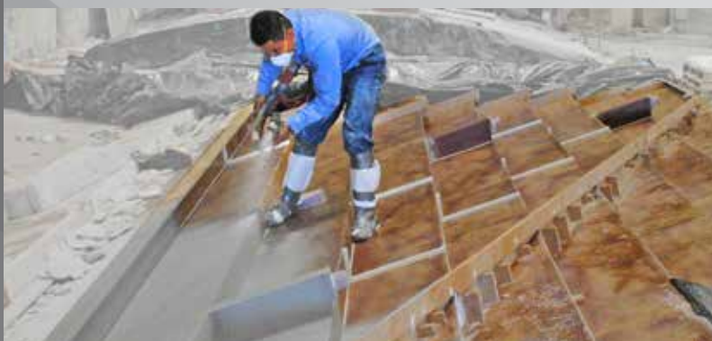
1 Two layers of a Forton™ VF-774 enhanced GFRC face mix are sprayed over form surfaces.
