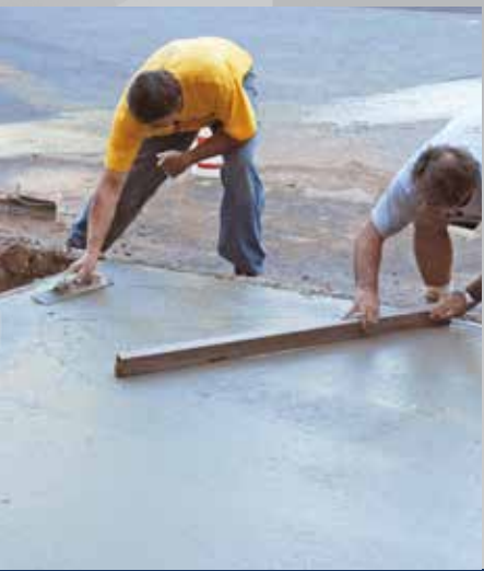
7 Concrete is screeded and color hardener is applied prior to stamping.
