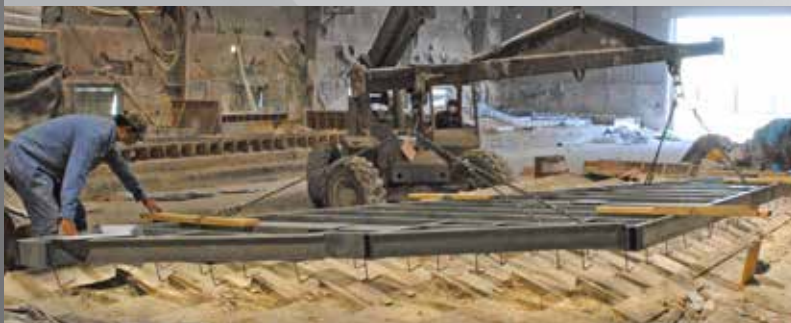
5 A structural steel frame is carefully lowered into place just above the wet concrete.
