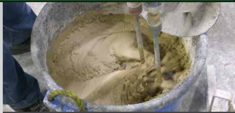
2 ECC Blended Mix™ is mixed and pigmented to a light tan color.
