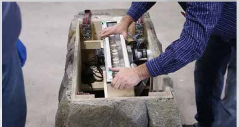
10 The top is sealed, and the faux fire generator is installed:
