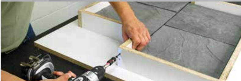
1 Mold box is built around stone pavers in a pattern.
